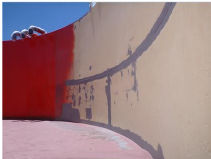
Surface preparation on tank wall
