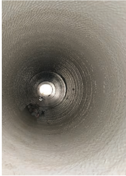
Fig. 4 (center and above): The finished, polyurea-lined pipeline was inspected and found to have rectified the historical problems with water intrusion and degradation at this site.
