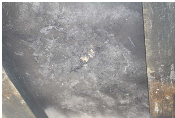
Post-blast exposed face heat/chem resistant layers
